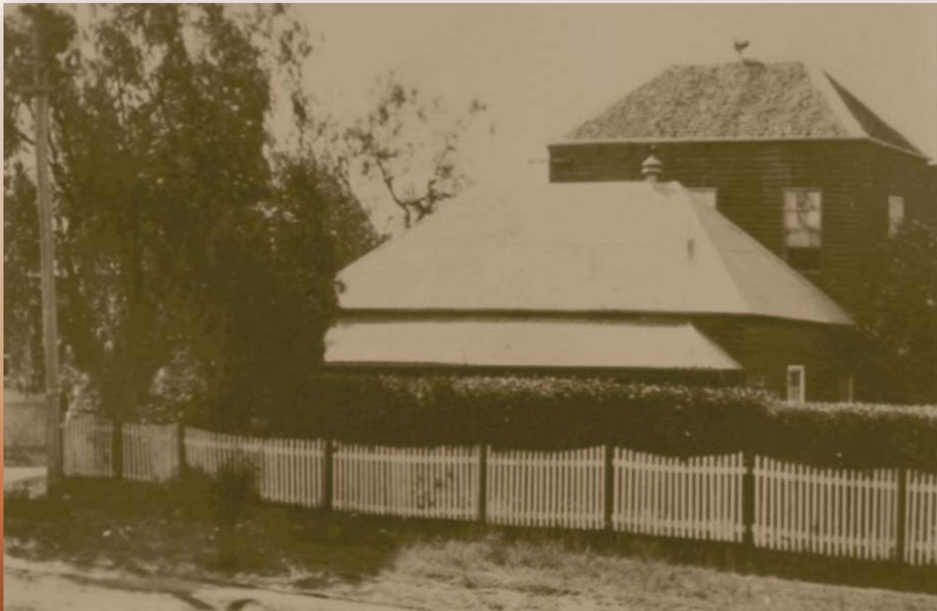
1884: Cottage purchased on the present site. Boarders' quarters added at the back
